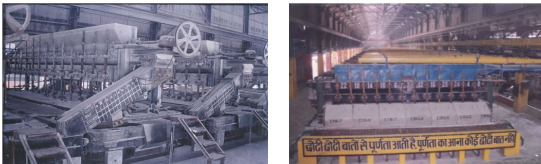
Figure 7. Renukoot smelter plant before and after modernization [2].
